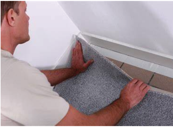
Laying a carpet
