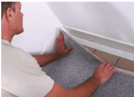
Laying a carpet
